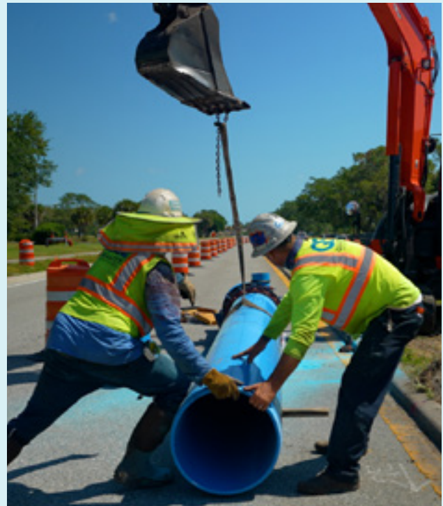
New water distribution main along NASA Boulevard, Dr. Martin Luther King Jr. Boulevard, and Apollo Boulevard
